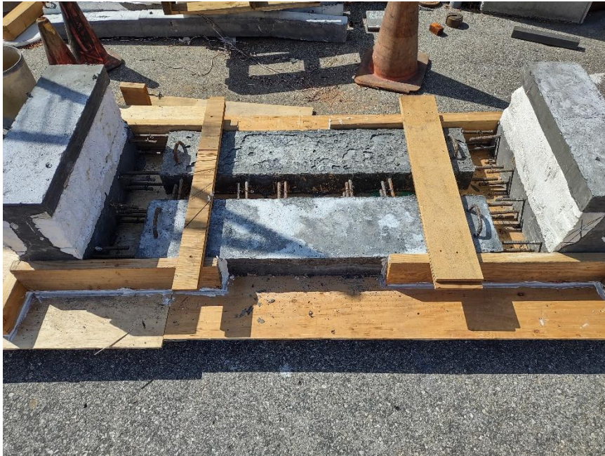
Fig. 3 Placement of panels and I-girders prior to joint pour
